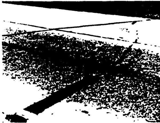
Fig. 3.2.4.6 — Diagonal crack
